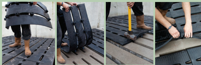
Picture Sequence shows the ease with which the Durapak Slatted Rubber Mat is positioned onto the slat
